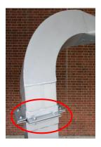
(C) Install Metal Discharge Hose (1) Clamp 12" Heavy Duty Fasten with (6) ½ x 1" bolts
